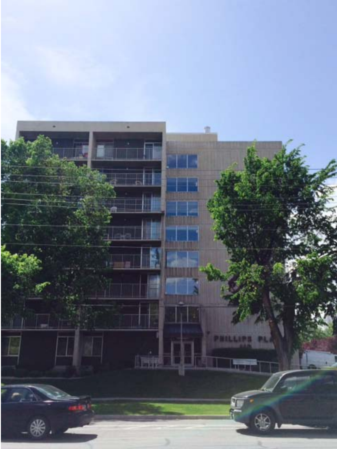
Looking towards the west at the front facade of the Phillips Plaza Apartment Building.
